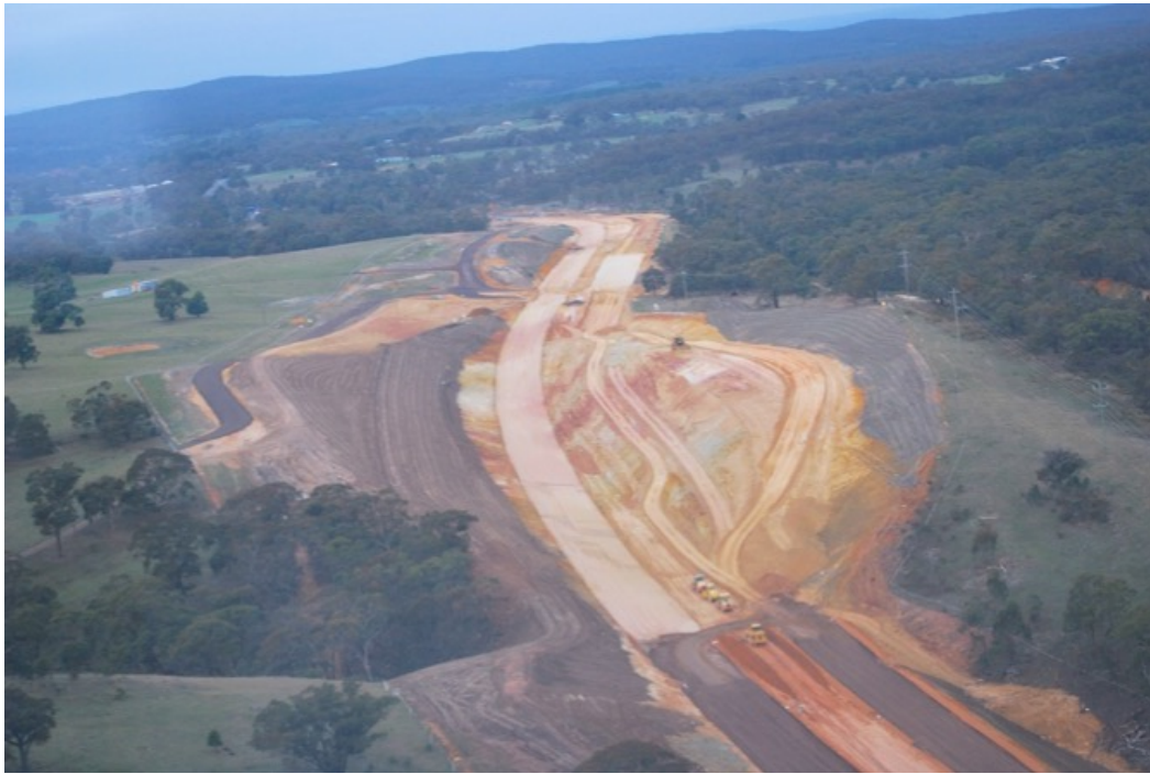
Figure 18. Box's Cutting on the Beaufort to Buangor section, 1.2 million cubic metres of Cut-and-Fill.
