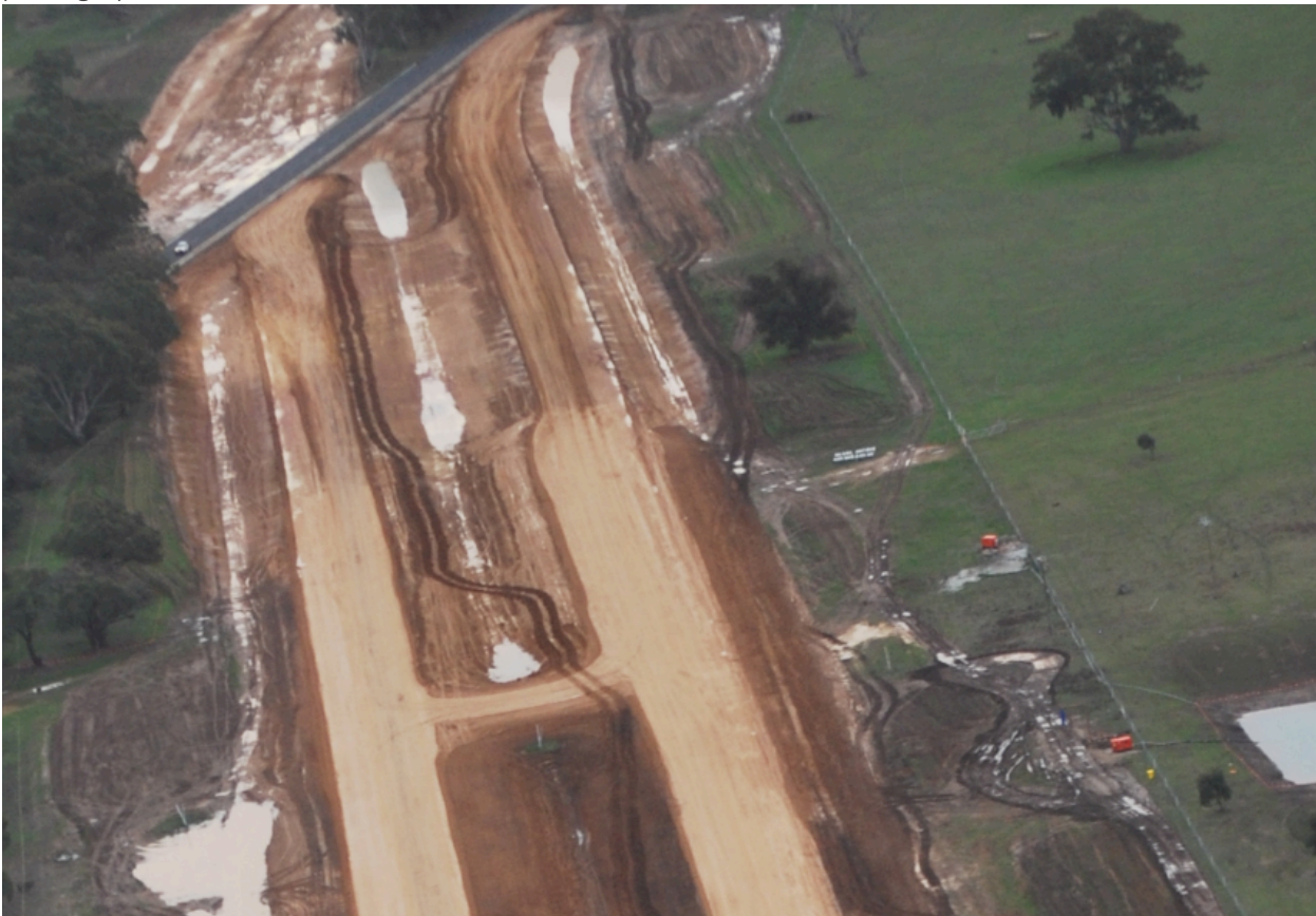
Figure 1. Road works for duplication at Buangor, 2015. The old highway runs across the top of the photograph.
